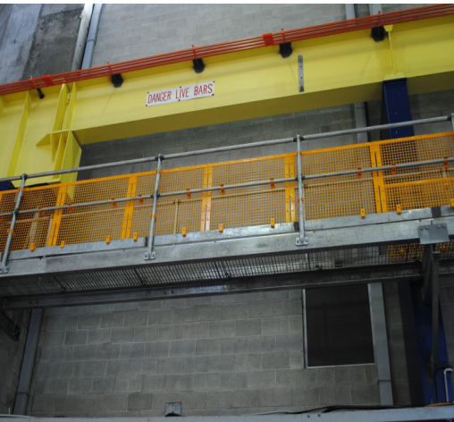
BLH Stop Drop™ Barricading installed on Walkways
